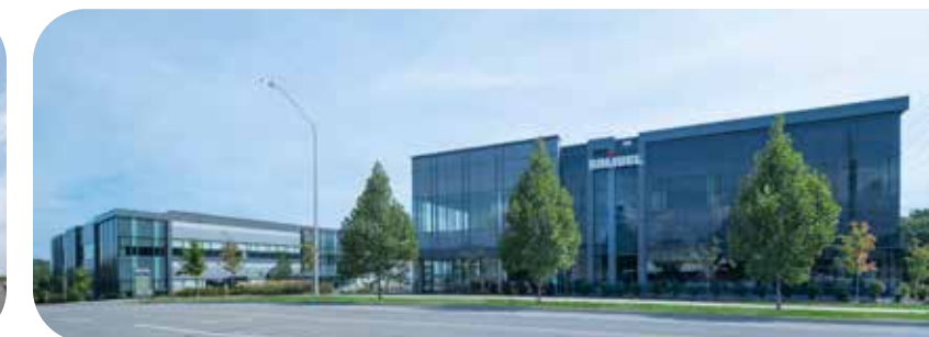
1900 & 1908 Ironoak Way, Oakville LEED Silver Certified
