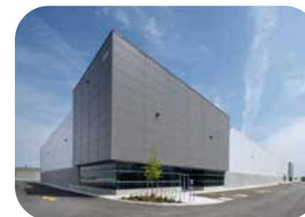
2510 & 2520 Royal Windsor Dr, Mississauga LEED Silver Certified
