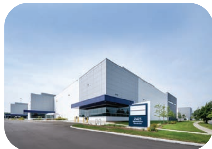
2425 & 2475 Meadowpine Blvd, Mississauga LEED Silver Certified
