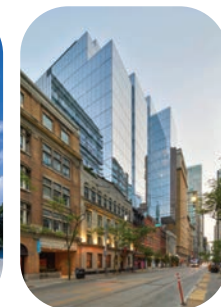
65 King St East, Toronto LEED Gold Certified
