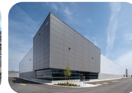
2510 & 2520 Royal Windsor Dr, Mississauga LEED Silver Certified
